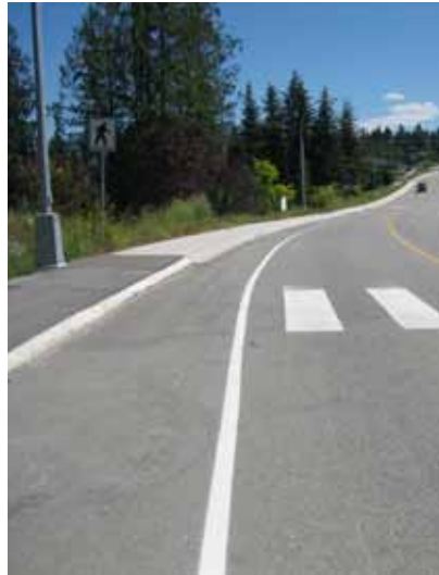
Bike lane and sidewalk
