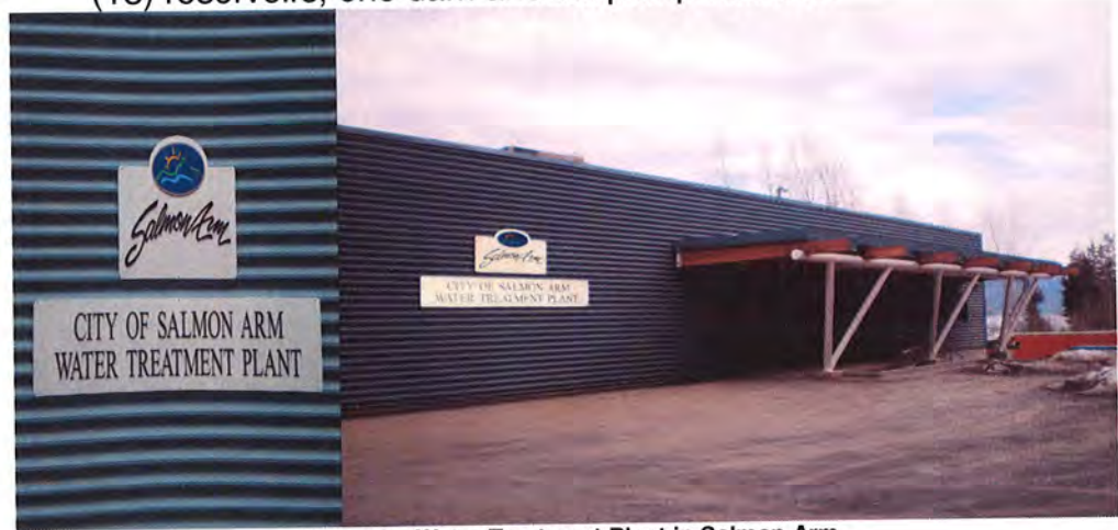
Figure 1 – Water Treatment Plant in Salmon Arm
