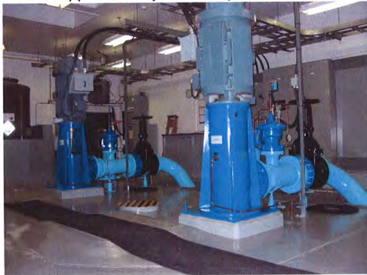
Figure 4 - Zone 1 Pumping Station Canoe
