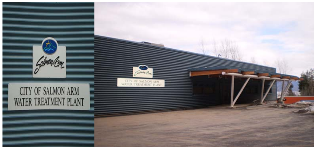
Figure 1 – Water Treatment Plant in Salmon Arm
