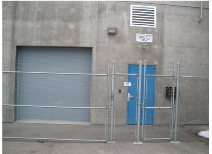
IR #3 Reservoir 251 Gleneden Road
