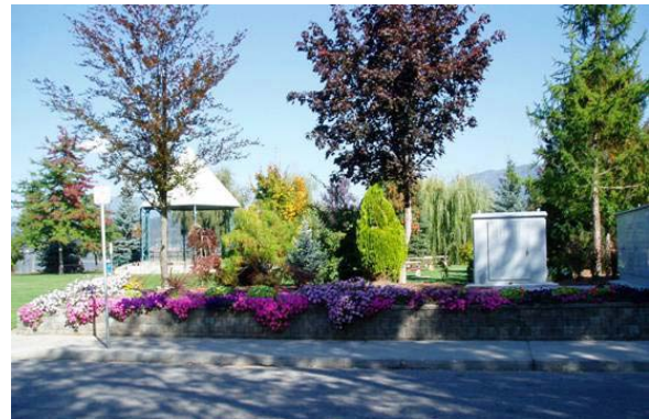
Wharf Street Lift Station
