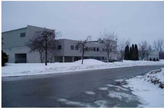
WPCC – After renovations
