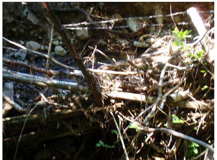
Mouzell, Segment 3, Obstruction Point 6
