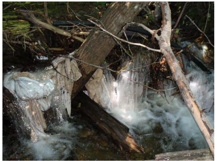
Mouzell, Segment 3, Obstruction Point 4
