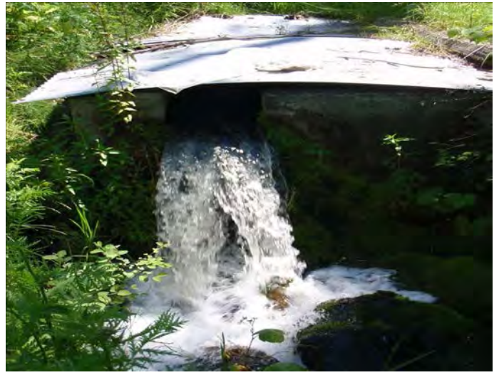
Rumball, Segment 3, Obstruction Point 3
