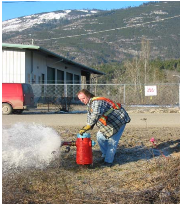
Figure 6 – Utilities Department operator flushing watermain as part of regular maintenance
