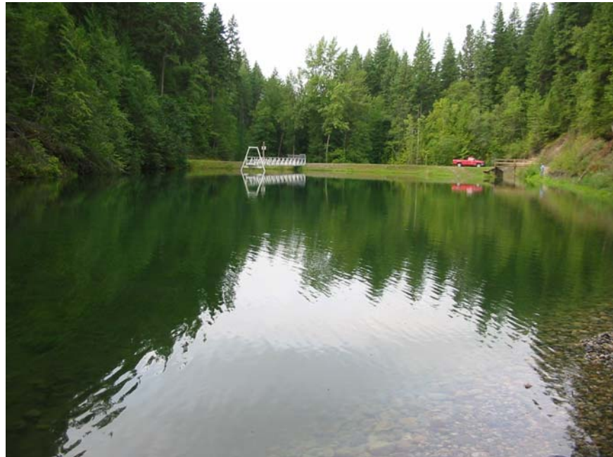
Figure 7 - Metford Dam (August, 2003)
