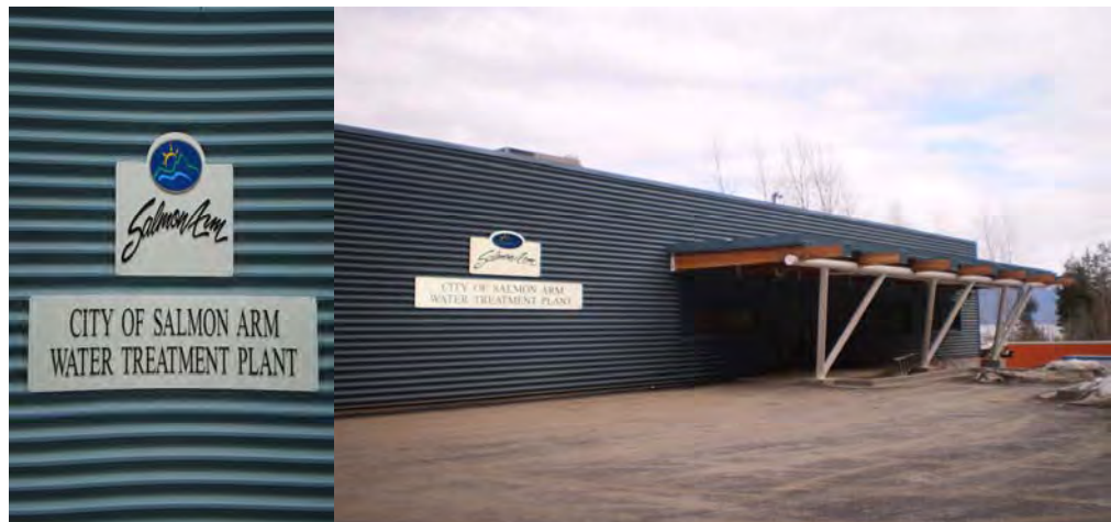
Figure 1 – Water Treatment Plant in Salmon Arm
