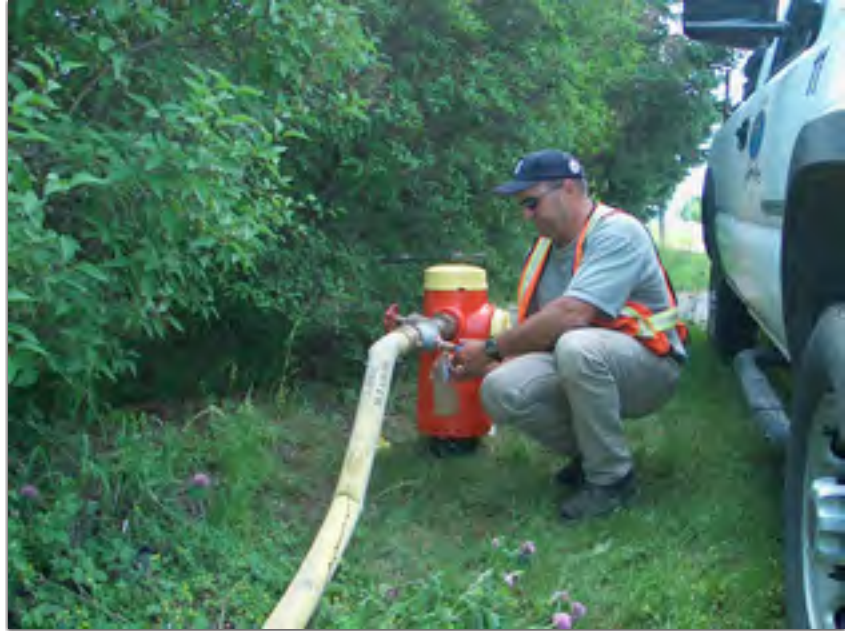
Figure 8 – Utilities Department operator flushing watermain as part of regular maintenance
