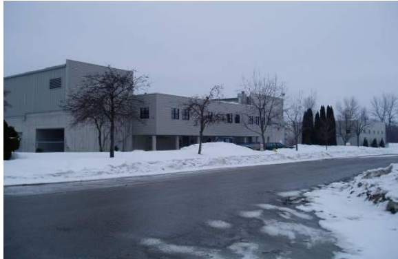
WPCC – After renovations
