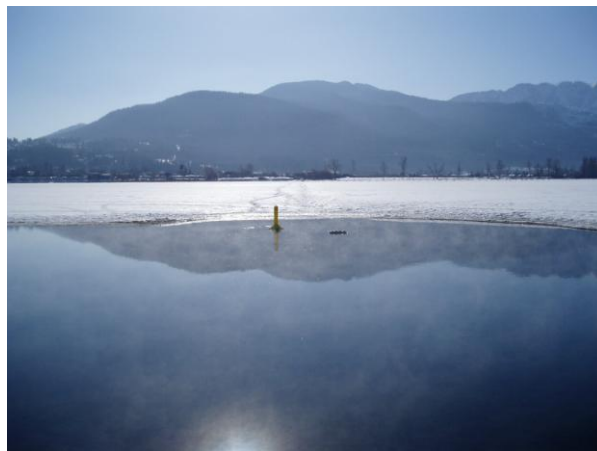
Outfall with marker buoy
