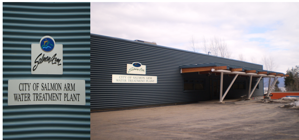
Figure 1 – Water Treatment Plant in Salmon Arm
