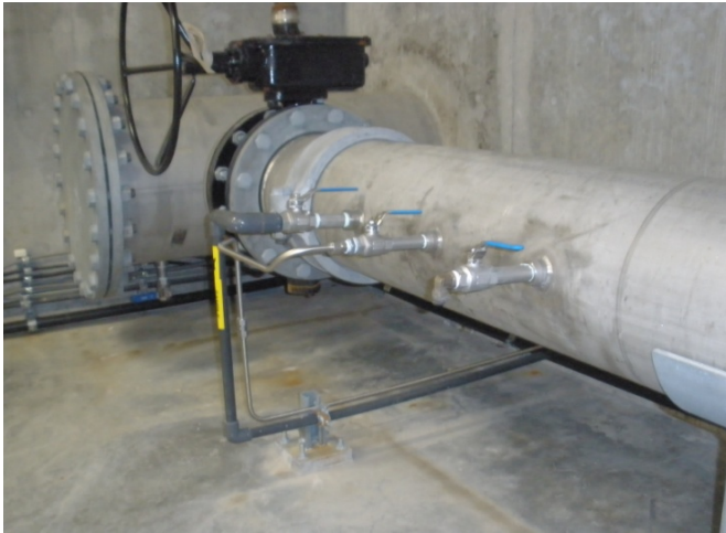
Water Treatment Plant 3751 Canoe Beach Dr NE
