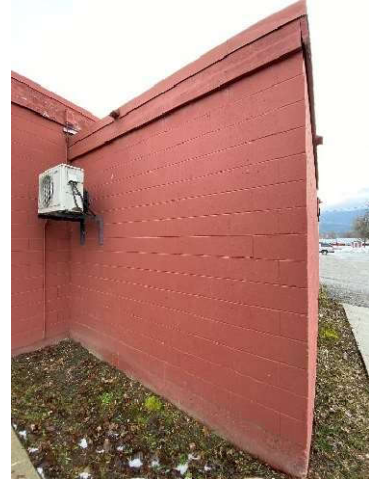
Photo 15: Typical condition of painted CMU.
