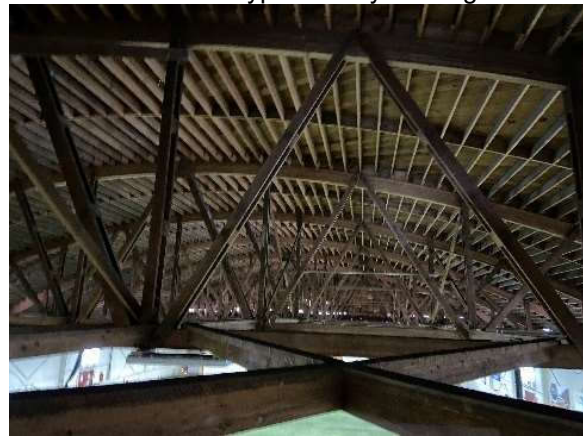
Photo 42: Typical bottom chord cross bracing.
