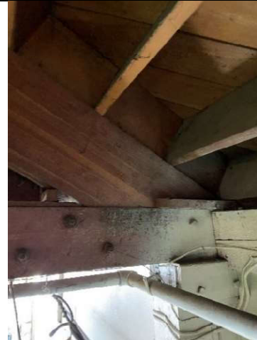
Photo 38.1: Truss bearing plate.
