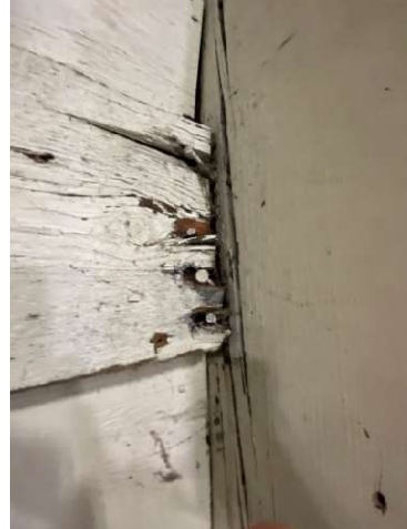
Photo 44: Strut to column connection.
