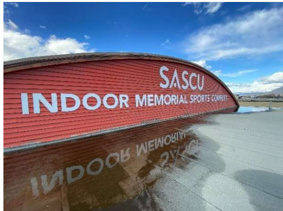
Photo 4: East arena flat roof.
