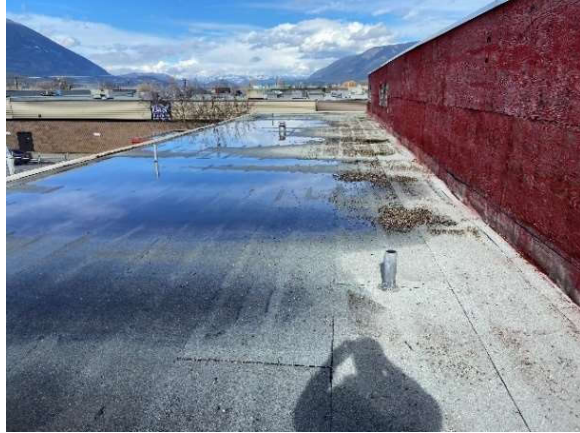
Photo 6: West addition upper roof typical condition
