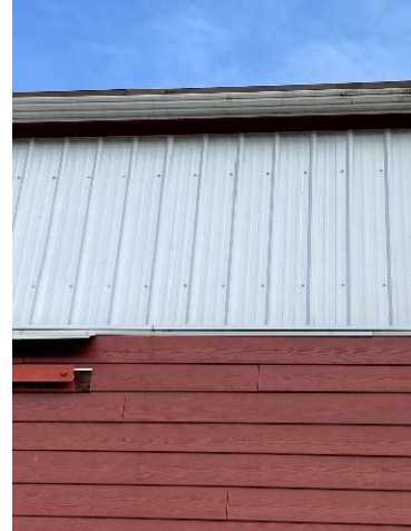
Photo 12: Vertical Metal Siding.
