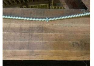
Photo 33: Typical condition of bottom chord. Note minor checking in 3rd lamnination.
