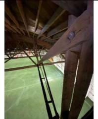
Photo 41: Typical sway bracing.
