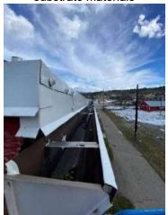
Photo 24: Aluminium gutters and flashing along south arena wall.
