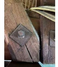
Photo 34: Typical splitting at web to chord connection.
