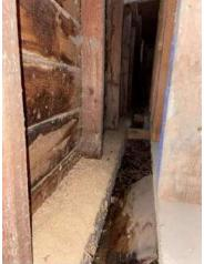
Photo 48: Typical infill studwall framing seen on left, bearing on bottom strut, partially below grade. Studs clad with horizontal lap siding. No sill plate observed. Moisture staining throughout.
