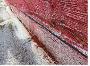
Photo 7: Microcracking, bond failure, and blistering observed.
