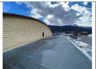
Photo 3: Flat roof at west end of arena. Ponding water observed.
