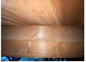
Photo 31:Observed splitting in rafter
