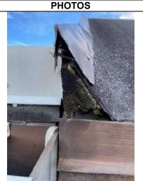
Photo 23: Gable flashing with deteriorated substrate materials
