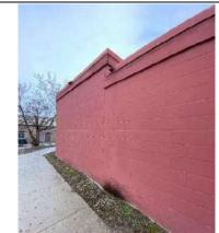
Photo 47: Typical condition of exterior CMU walls.
