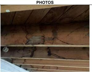
Photo 30: Water staining observed on arena rafters.
