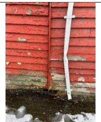
Photo 9: Ceder lap siding severely deteriorated within 48" of grade.
