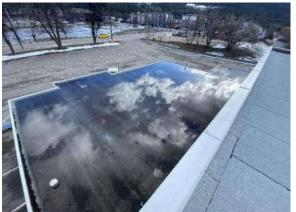
Photo 5: East addition lower roof flooded.
