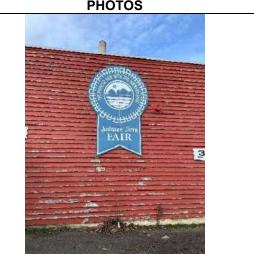
Photo 8: Typical condition of ceder lap siding.
