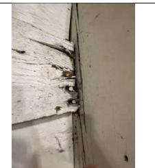
Photo 44: Strut to column connection.
