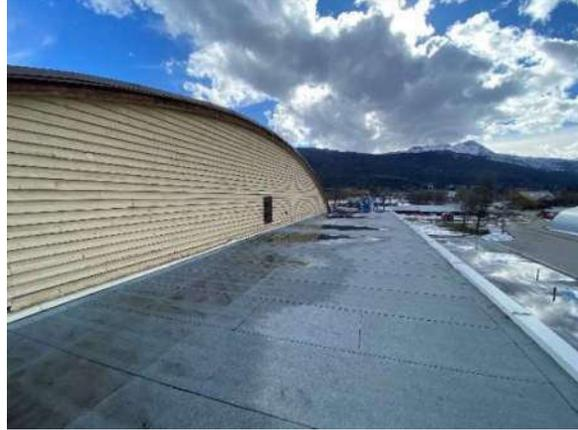
Photo 3: Flat roof at west end of arena. Ponding water observed.
