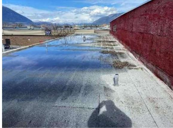
Photo 6: West addition upper roof typical condition
