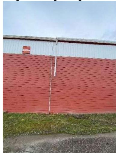
Photo 11: Typical condition of Hardi-plank lap siding.
