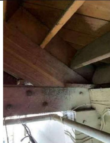
Photo 38.1: Truss bearing plate.
