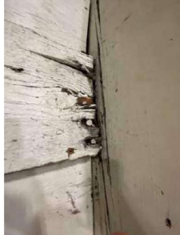
Photo 44: Strut to column connection.
