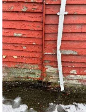
Photo 9: Cedar lap siding severely deteriorated within 48" of grade.
