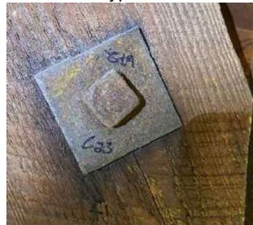
Photo 39: Typical surface corrosion on connection hardware.
