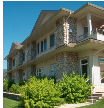
The use of local material such as stone on this building helps to create a strong identity and character in the City Centre
