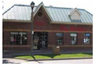
A good example of an interesting roof and a coordinated façade
