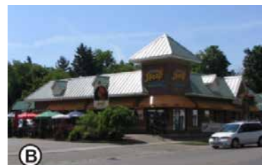
Photos A and B illustrate good examples of treatments for commercial building entrances, signs, and roof design
