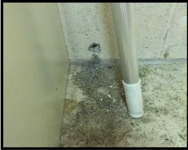
Asbestos-containing vermiculite insulation present as debris in the Back Storage (Loc. 17)
