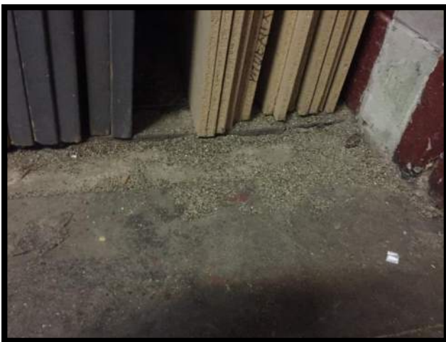
Asbestos-containing vermiculite insulation present as debris in the Workshop (Loc. 18)
