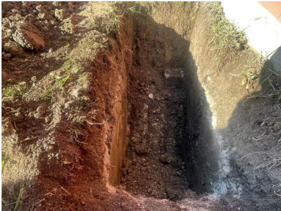
Photograph 6 – TP2 Exposed the edge of existing footing.
