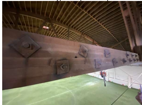
Photo 37: Typical bottom chord splice.
