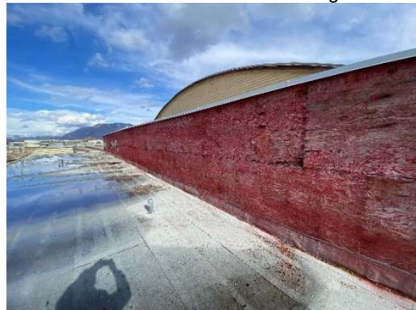
Photo 13: Typical condition of plywood sheathing.
