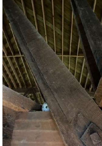
Photo 35: Web member with checking along entire length.
