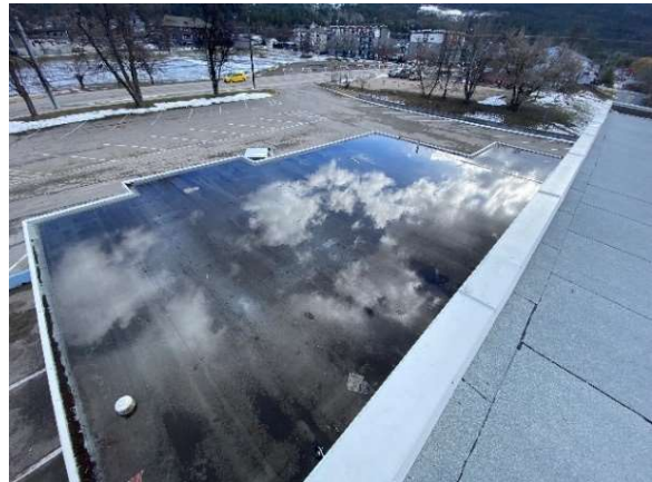
Photo 5: East addition lower roof flooded.
