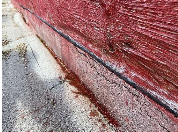
Photo 7: Microcracking, bond failure, and blistering observed.
