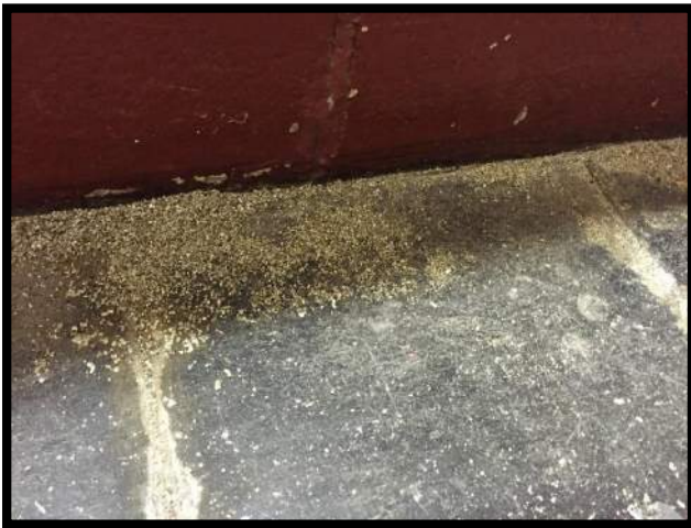
Asbestos-containing vermiculite insulation present as debris in the Back Hallway (Loc. 15)
