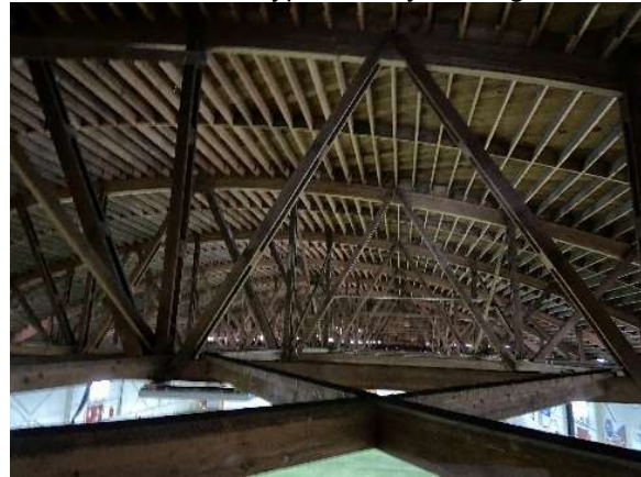
Photo 42: Typical bottom chord cross bracing.
