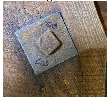
Photo 39: Typical surface corrosion on connection hardware.
