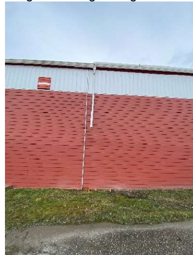
Photo 11: Typical condition of Hardi-plank lap siding.
