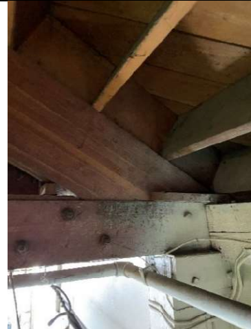
Photo 38.1: Truss bearing plate.
