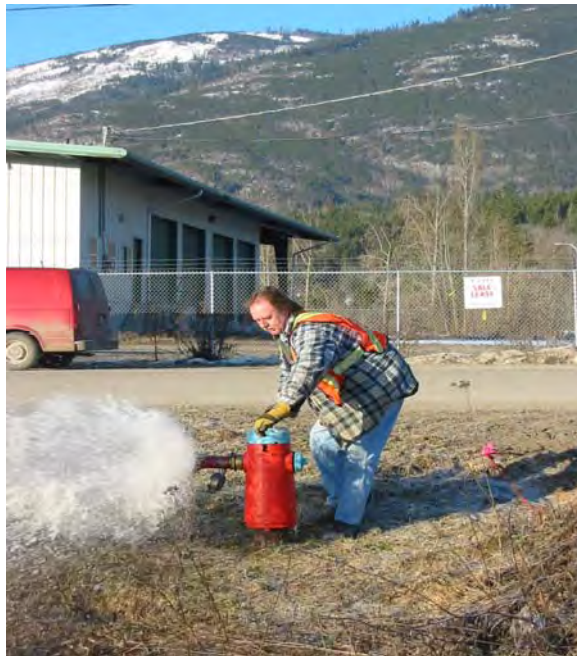
Figure 8 – Utilities Department operator flushing watermain as part of regular maintenance
