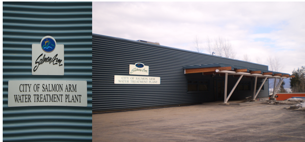
Figure 1 – Water Treatment Plant in Salmon Arm
