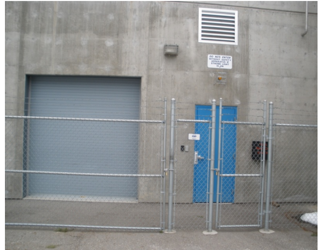
IR #3 Reservoir 251 Gleneden Road
