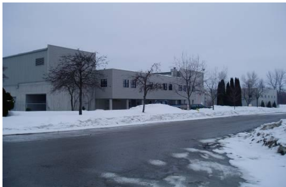
WPCC – After renovations
