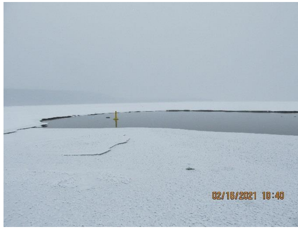
Outfall with marker buoy
