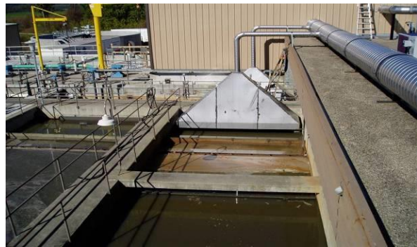
Primary Sedimentation Tanks
