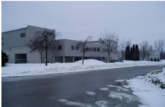
WPCC – After renovations
