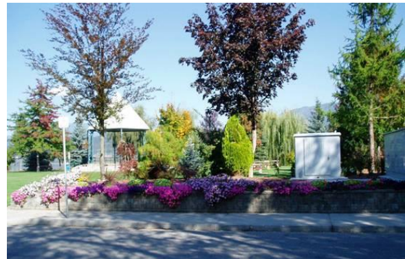
Wharf Street Lift Station
