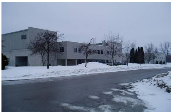
WPCC – After renovations
