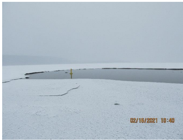
Outfall with marker buoy
