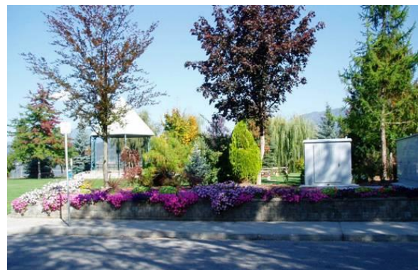
Wharf Street Lift Station
