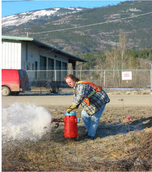
Figure 9 - Salmon Arm operator flushing watermain as part of regular maintenance
