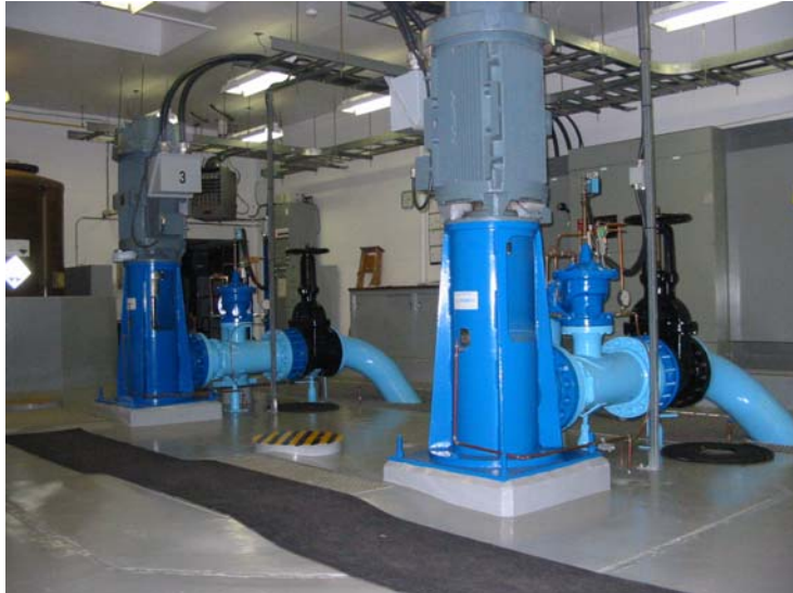
Figure 4 - Zone 1 Pumping Station Canoe
