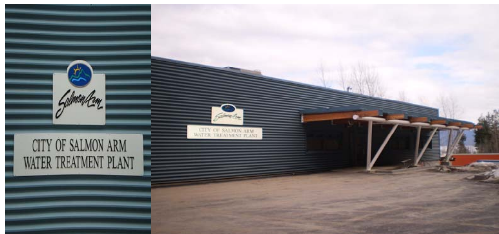
Figure 1 – Water Treatment Plant in Salmon Arm
