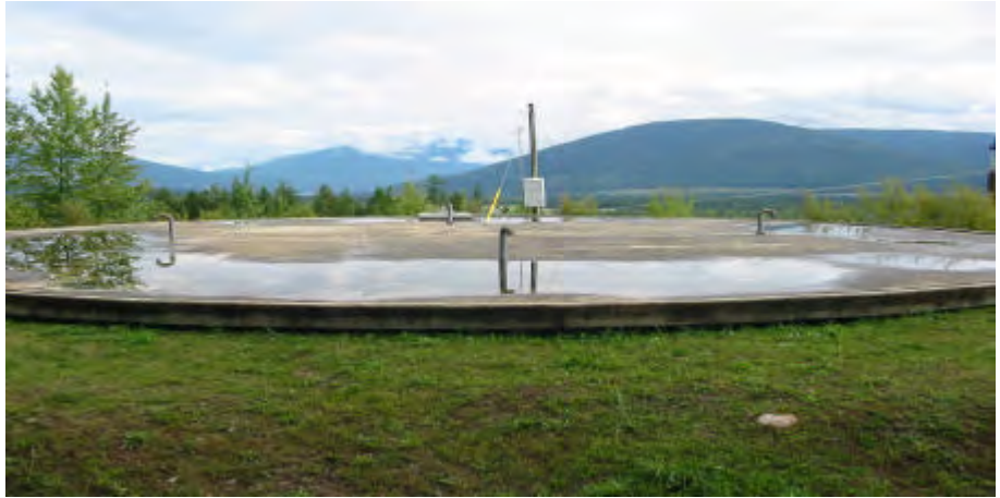
Figure 5 – Zone 5 Water Storage - 2020 Water Reservoir on 40 th Street SE
