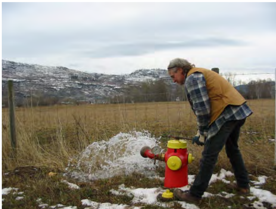
Figure 9 - Salmon Arm operator flushing watermain as part of regular maintenance.
