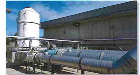
Foul air extraction and odour scrubbers can significantly reduce odour release to the atmosphere
