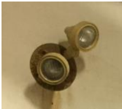
Figure 19: Twin Head Remote Emergency light
