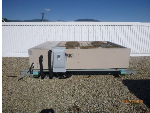
Figure 71 AHU - 2 Condenser
