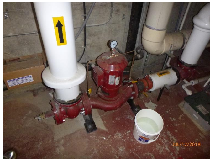
Figure 65 Boiler Pump
