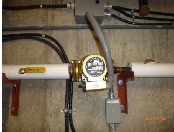
Figure 44 DHWR Pump
