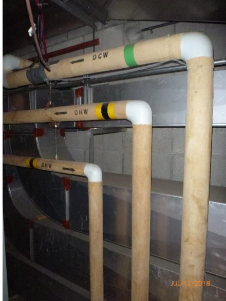
Figure 42 Domestic Water Pipework
