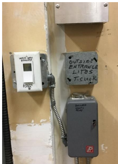
Figure 25: Existing exterior lighting controls and relays
