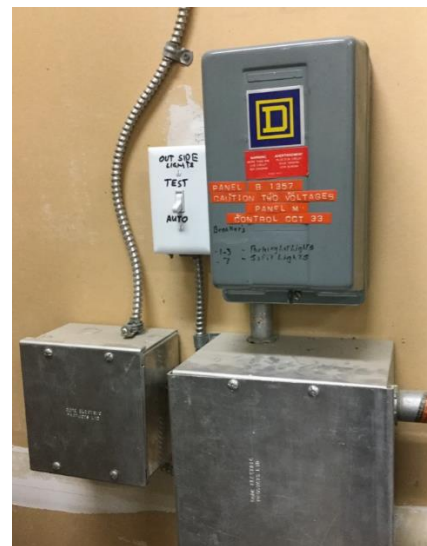
Figure 25: Existing exterior lighting controls and relays
