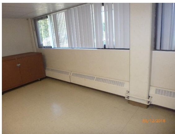
Figure 68 Radiant Panes and Hydronic Base Board Heaters
