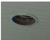
Figure 15: Recessed Lensed Downlight
