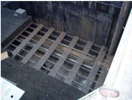
WPCC Trickling Filter Media Replacement
