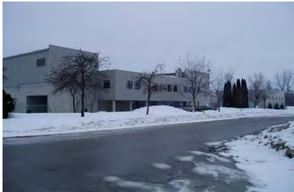
WPCC – After renovations
