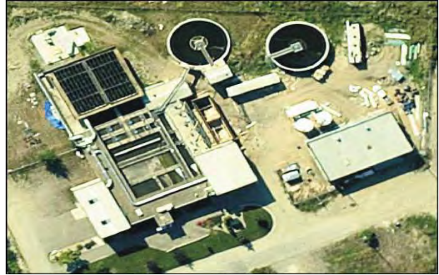
Aerial Photo Stage IIIB prior to Landscaping
