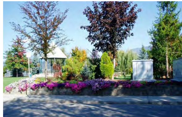
Wharf Street Lift Station
