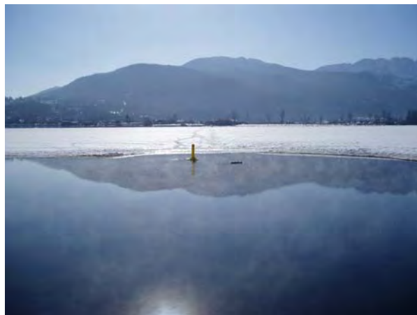
Outfall with marker buoy
