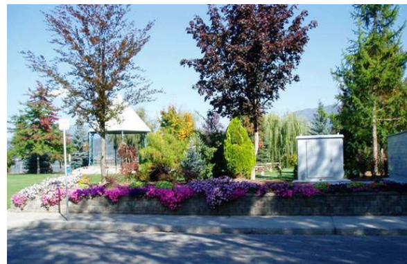
Wharf Street Lift Station
