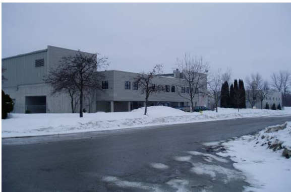
WPCC – After renovations
