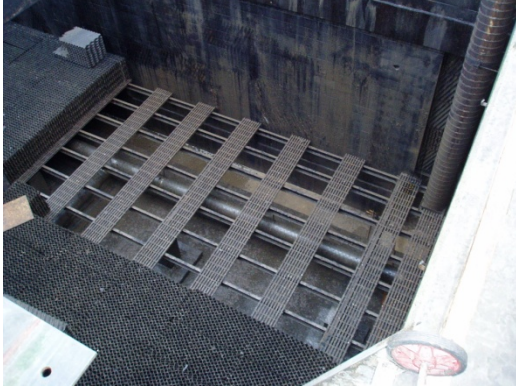
WPCC Tricking Filter Media Replacement
