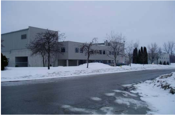
WPCC – After renovations
