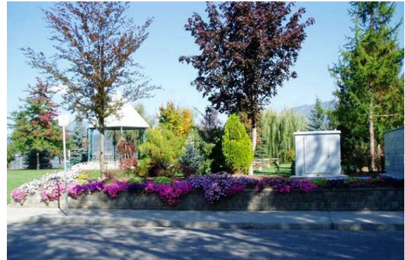
Wharf Street Lift Station
