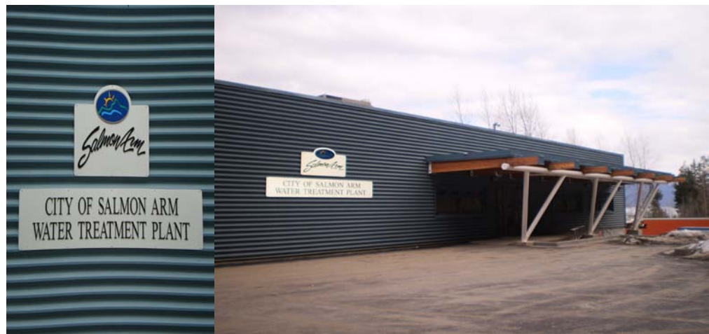
Figure 1 – Water Treatment Plant in Salmon Arm
