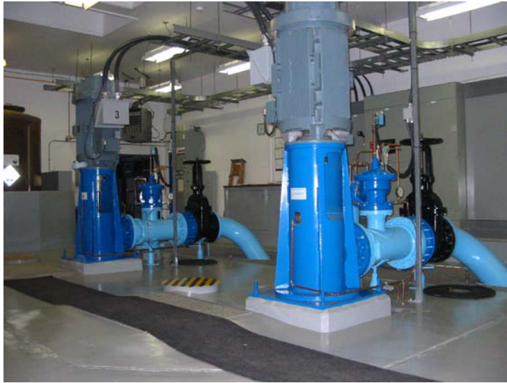
Figure 4 - Zone 1 Pumping Station Canoe
