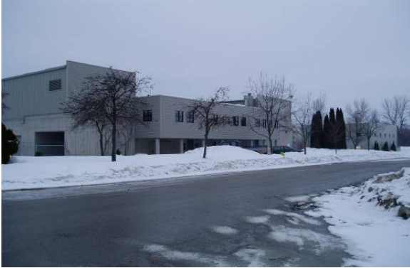
WPCC – After renovations
