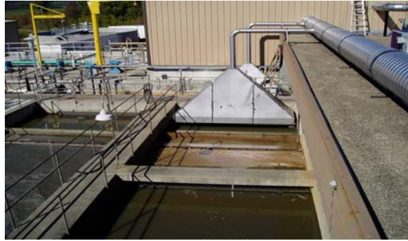
Primary Sedimentation Tanks
