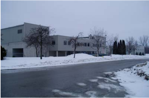
WPCC (after Renovations)
