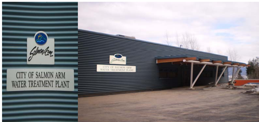
Figure 1 – Water Treatment Plant in Salmon Arm
