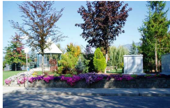
Wharf Street Pump Station
