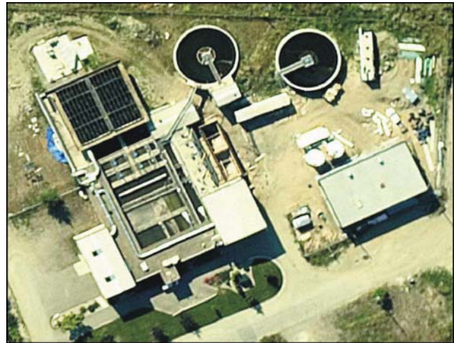
Aerial Photo Stage IIIB prior to Landscaping
