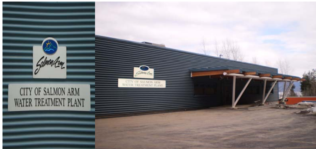
Figure 1 – Water Treatment Plant in Salmon Arm
