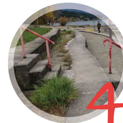
Retaining Walls and Stairs
