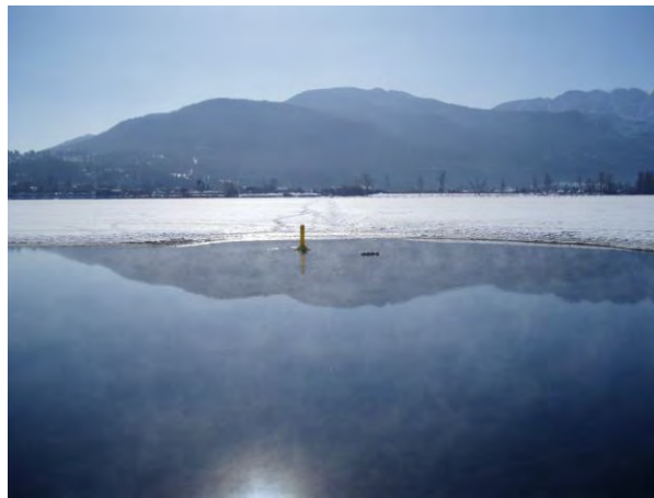
Outfall with marker buoy
