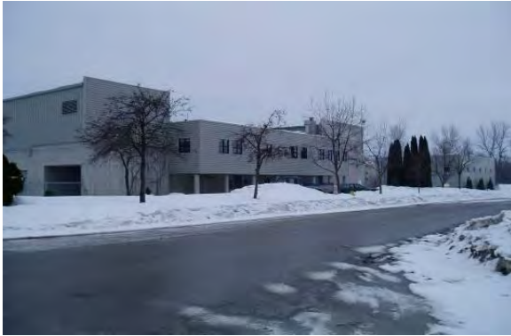
WPCC – After renovations
