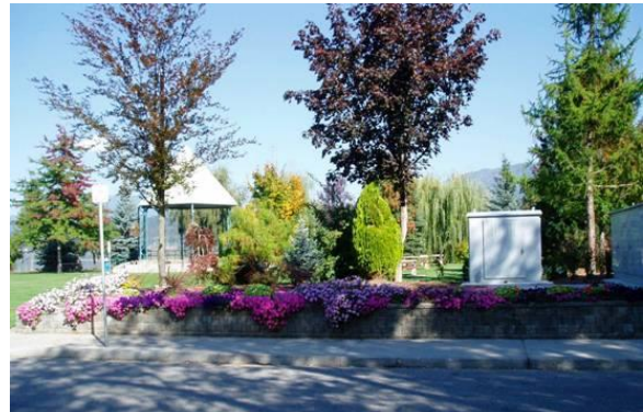
Wharf Street Lift Station
