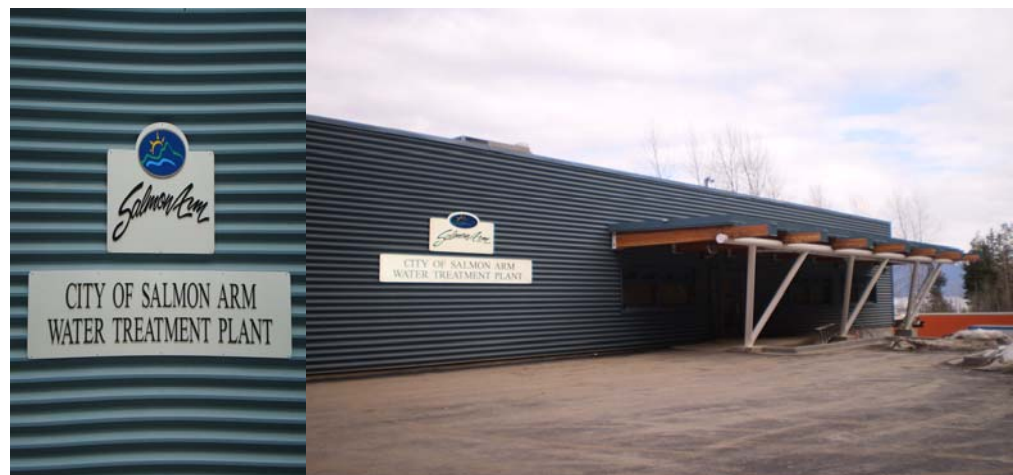
Figure 1 – Water Treatment Plant in Salmon Arm
