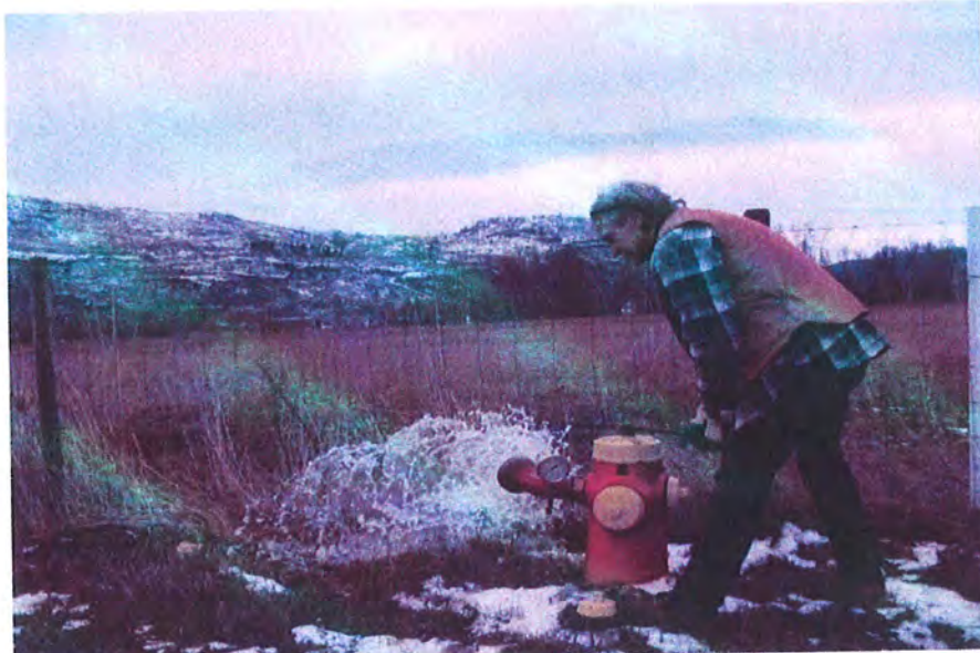
Figure 1 – Utilities Department operator flushing water main as part of regular maintenance
