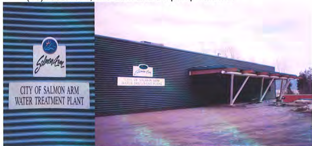
Figure 1 – Water Treatment Plant in Salmon Arm
