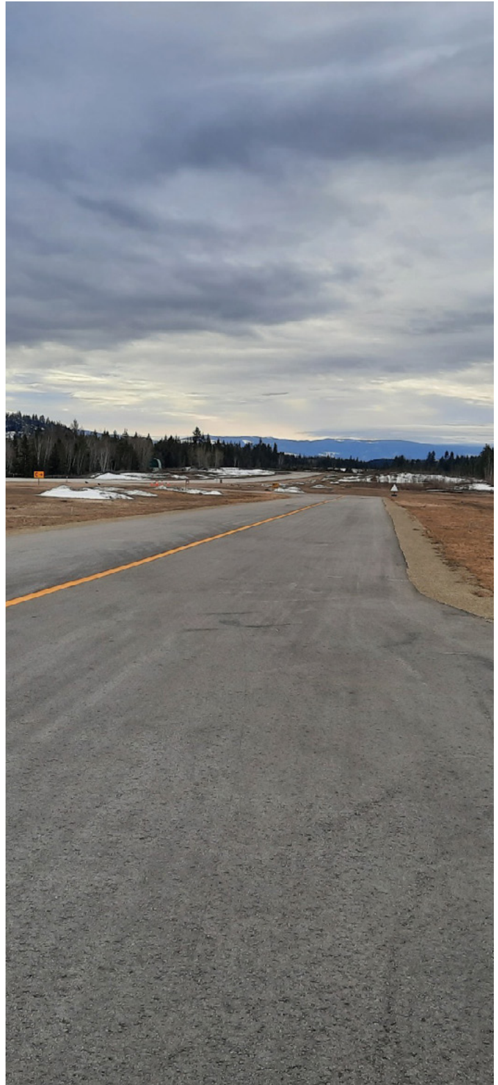
Taxiway Charlie - Shuswap Regional Airport
