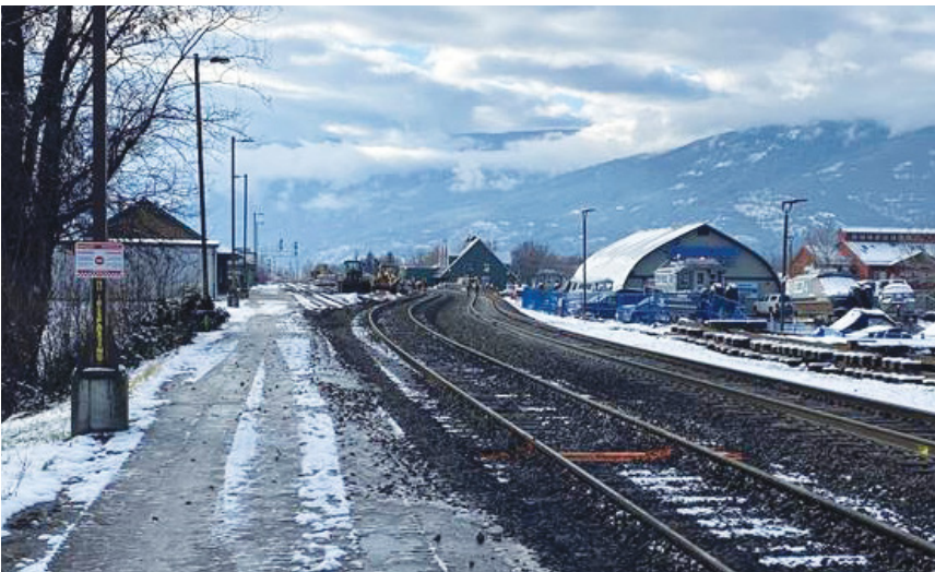
Track detour for Ross Street underpass
