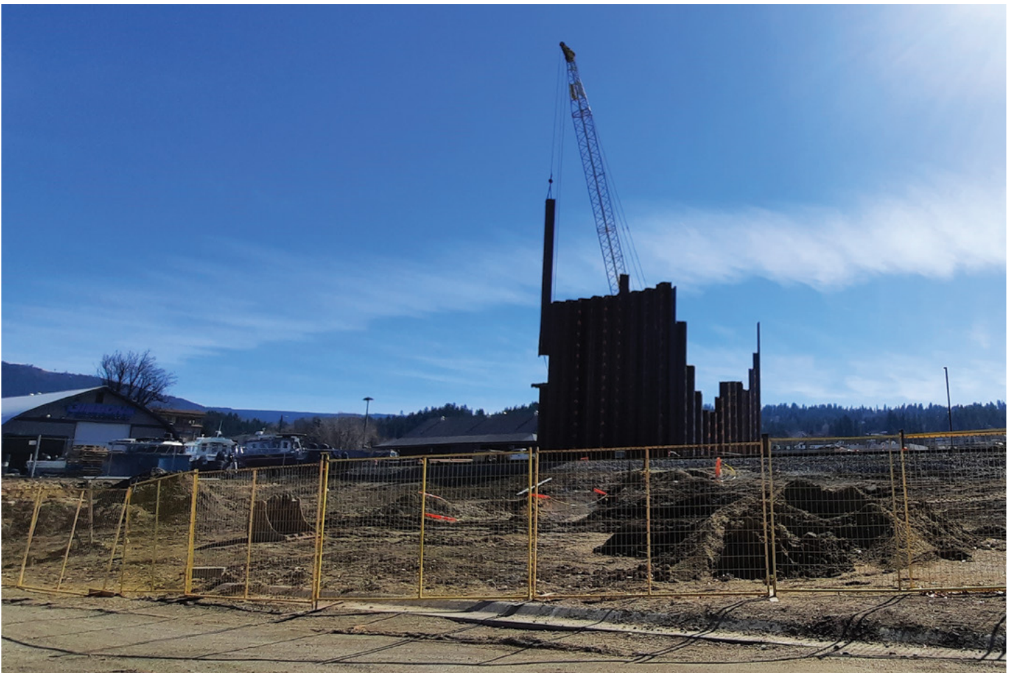
Steel plate shoring installation - Ross Street Underpass
