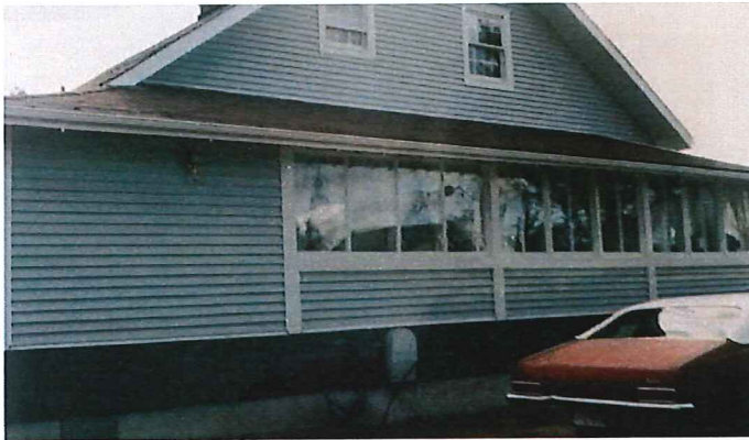
Side of house AFTER renovations
