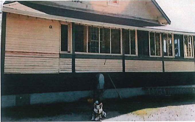
Side of house BEFORE renovations
