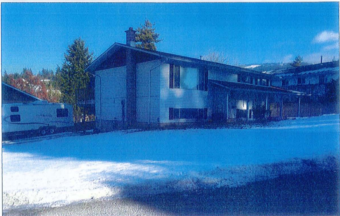
View east of subject property from 21 Street NE.
