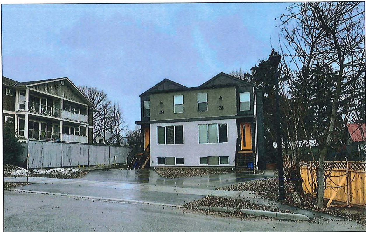
View of subject parcel southeast from 4 Street SE.
