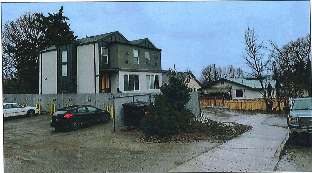
View of subject parcel northwest from 4 Street SE.
