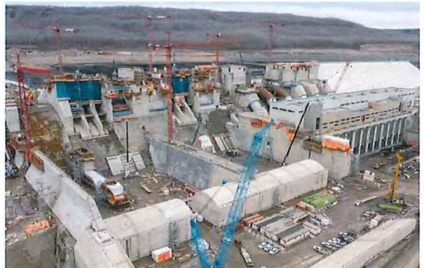
This aerial view shows Site C's spillways, penstocks, powerhouse and operations building for BC Hydro's third dam along the Peace River. Photo courtesy of Site C Team, BC Hydro.
