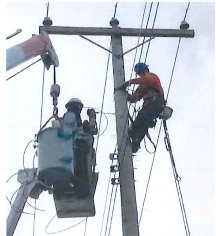
BC Hydro crews restoring electrical infrastructure in the Village of Lytton in January 2023. Photo courtesy of Clay Rhodenizer
