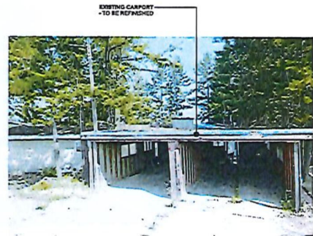
EXISTING CARPORT - TO BE REFINISHED
