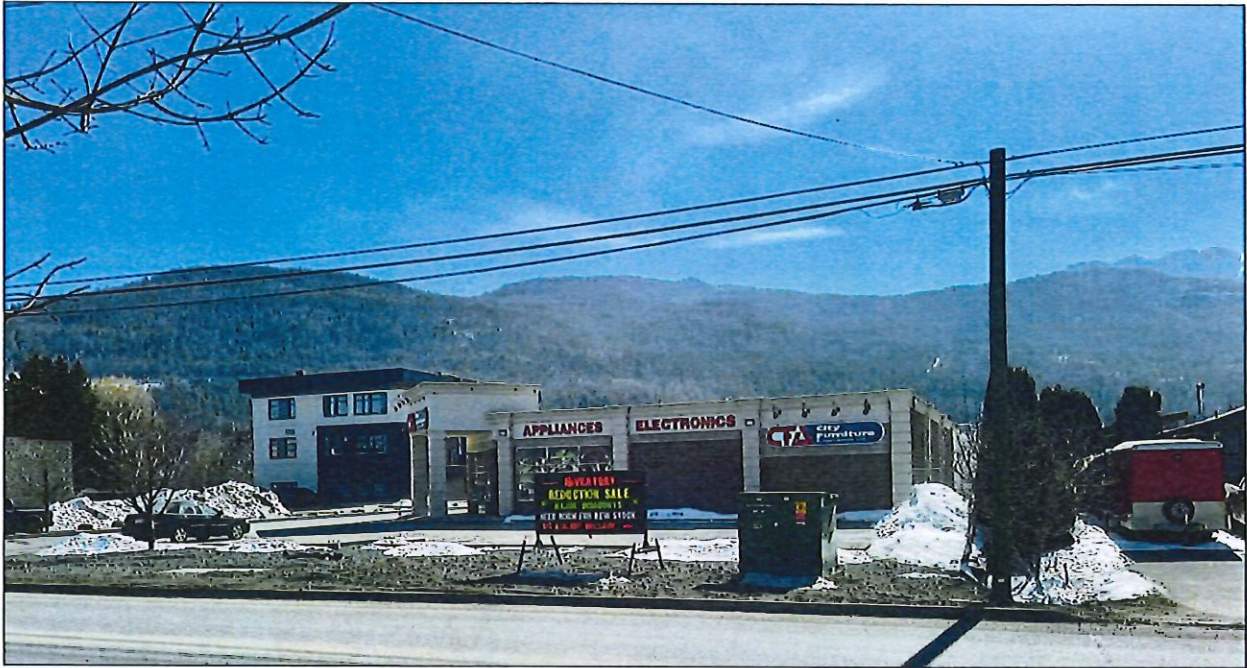
View of subject property southeast from 10 Avenue SW.
