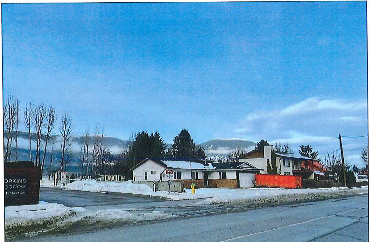
View of subject parcel northwest from 10 Street SW.
