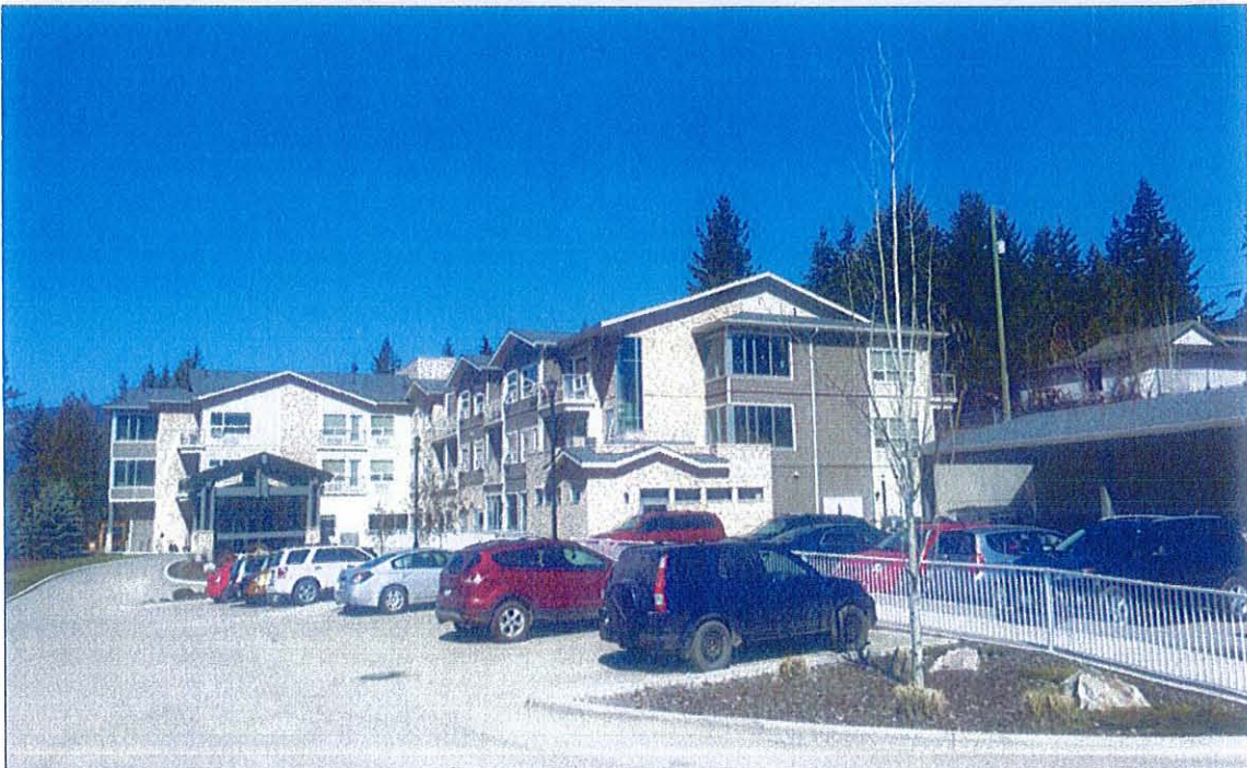
View north of Andover Terrace.
