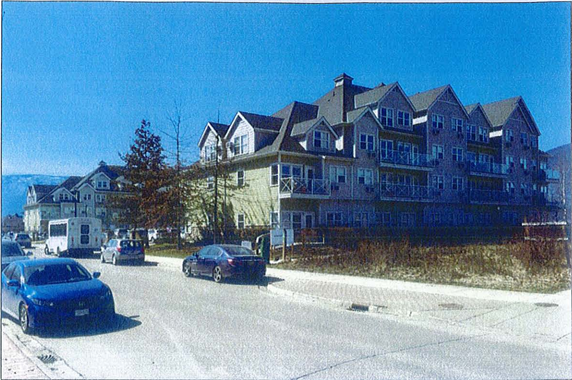
View to the north-west of Lakeshore Manor.
