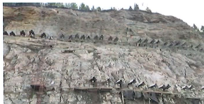
Installing protection for anchors.
