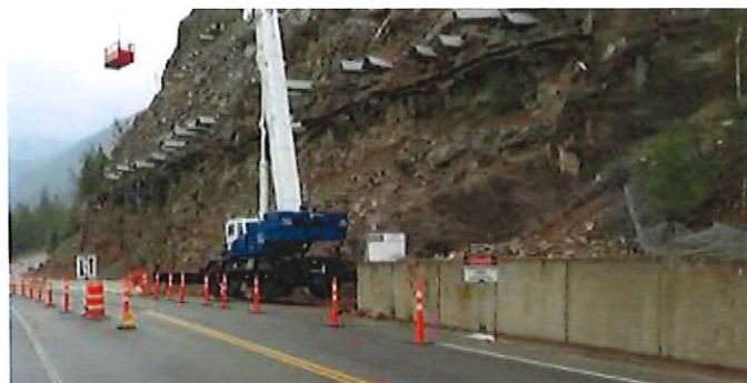
Crane being used to access the slope.
