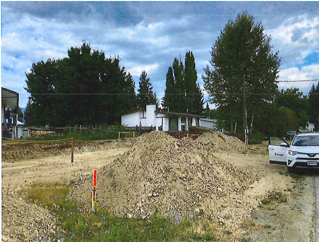
View of subject parcel looking northwest from 28 Street SE.
